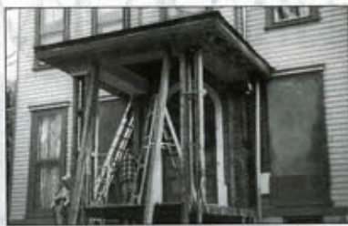
The new front porch, in progress.
