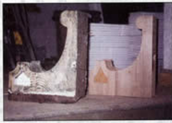
A restored bracket, left, and a new one, right, made to look like the old.
