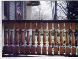
Period balusters were painted to match the historic colors chosen for the house.
